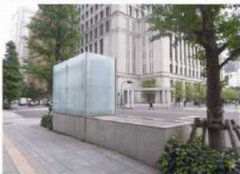
Ventilation / Fire Exhaust
